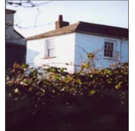
With noteworthy exceptions at each end of the village street, continuous terraces are not a common form, so that side or end walls figure prominently in most views along it. The majority are gabled, but few views don't include at least one that's hipped. This one, at Church Cottage (above right), shows hips in their most attractive form, with their original 'mitred-slate' finish still preserved
