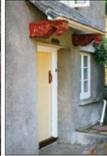
The corbels supporting the porch on this 19 th century looking cottage (left) probably date from the late 17 th century and suggest the cottage actually has much earlier origins than its appearance would have us believe.
