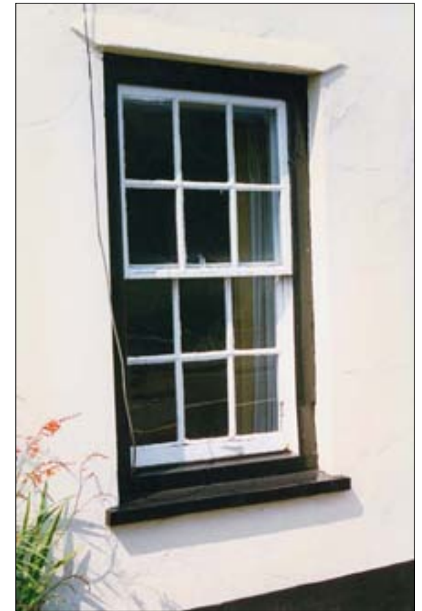
One of the many timber sash windows introduced in the 19 th century which contribute so very much towards Yealmpton's authentic historic character
