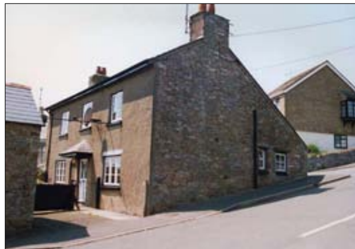
Quarried locally, grey limestone with bluses of pink or brown is the dominant material for wall construction, although more often than not it has been purposefully hidden beneath render to create a more 'polite', less rustic, appearance, particularly on principle elevations (above).
