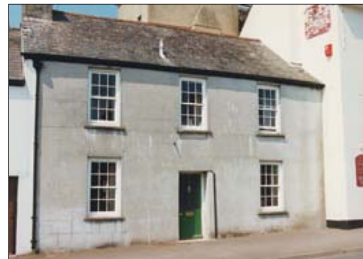
One of several cottages in the Area dating from the 16 th or 17 th centuries that have had their 'vernacular cottage' style transformed to 'polite house' when refronted with sashes and ashlar-lined render in the 19 th century – which are here admirably preserved. Along with its terraced neighbours, the house occupies one of a series of plots probably laid out in medieval times as part of a planned settlement – which at this end had a broad market place that included the land now occupied by the Post Office and Health Centre blocks. While none in the terrace are listed, it nevertheless makes a valuable contribution towards the interest and character of the Area.
