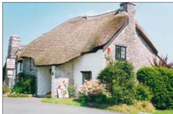
Probably the most picturesque building in the Conservation Area, 'Old Mother Hubbards' is one of the few to display a genuine vernacular style and character with its irregular form and appearance. The painting of some of its stonework is unusual in the Area, while its thatched roof is one of only three that survive to impart an 'ancient settlement' feel to the village scene. Its simple flush ridge is entirely in keeping with local traditions.
