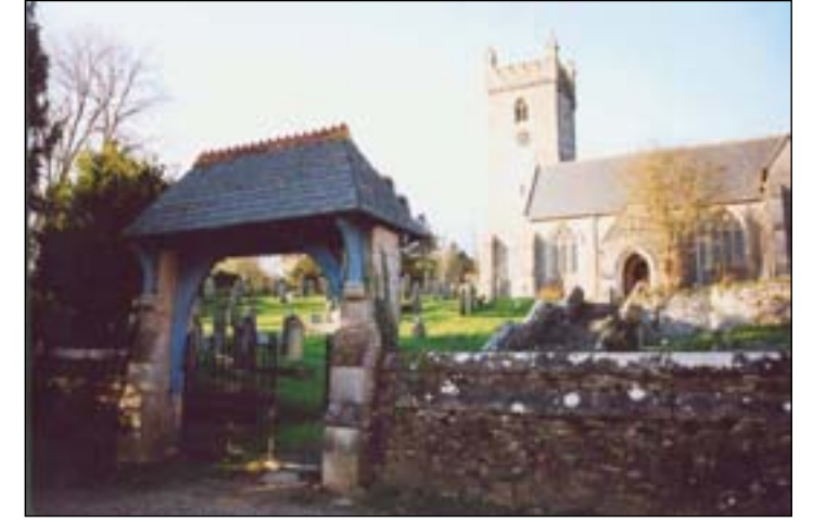
The Church and the Steps leading up to its porch are listed, but the Lychgate that's listed is the other one, shown on the front cover.
