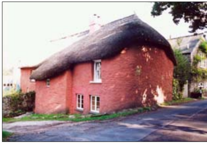
On roofs, which are mostly gabled, slate is the dominant cladding material, although the prominence of buildings clad in either sheet materials or thatch might suggest otherwise. Quay Cottage (above) was, and still is, one of these because it was clad in sheets and only recently celebrated its return to thatch.
