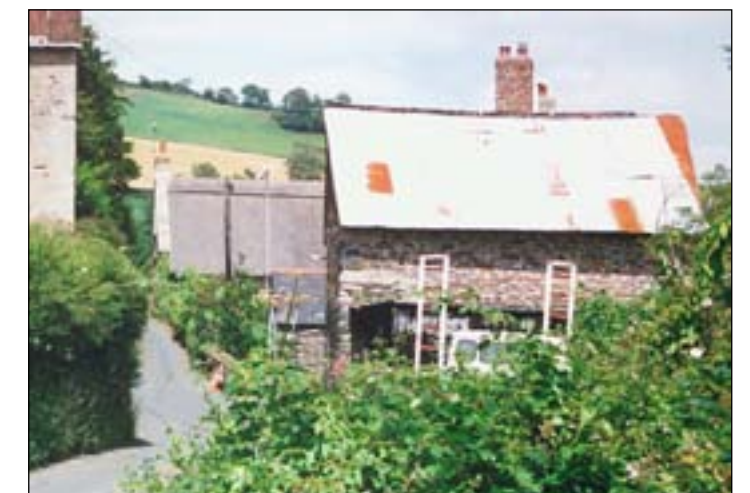
The mill building and the store on the opposite side of the lane are reminders of a more industrial past and create a very distinctive edge, and 'entrance' to the creek-side group.
