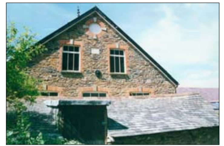
Although characterising the window openings of the later paper mill buildings in a quite distinctive way (above), brick has otherwise been used only sparingly throughout the hamlet. The same is true of slate hanging, although old photographs show this was formerly more in evidence.
