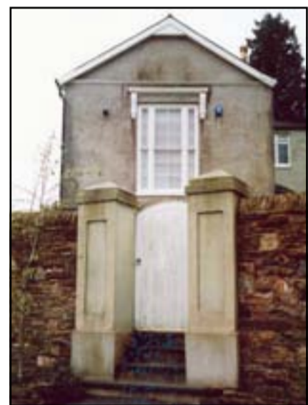
Proving the point that rendered surfaces can be a positive source of character, that applied to Tuckenhay House preserves both the patina and authenticity of its age by remaining true to its original, unpainted finish.
