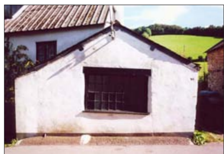
One of the very few buildings whose exposed stonework has been masked beneath render. Nevertheless, the building's old display window and slate verges add much interest and character to this part of the Area even though its not a listed building.
