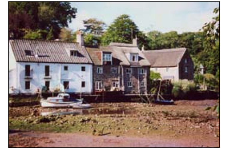
Rising directly off the revetments, this terrace of cottages dominates what is now a picturesque and tranquil scene. Nevertheless, they might hold the secret of a less than tranquil past if, like Riverside to their right, they also had some former storehouse use. This would certainly help explain their unusual siting, and support the view that the Wash was the location of Tuckenhay's earliest quays, possibly constructed in medieval times to service Cornworthy Priory via the ancient zigzag path to Cornworthy Cross.
