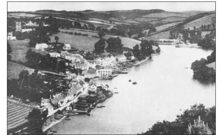
Newton Ferrers 1910 showing all of the conservation area
