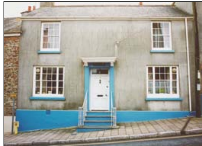
The majority of rendered surfaces are smooth and plain, but few still have their original unpainted (or simply lime-washed) finish. This house in Brownston Street is one that does, along with the original 'ashlar-lining' intended to give the appearance of finely-jointed, 'up-market' masonry.
