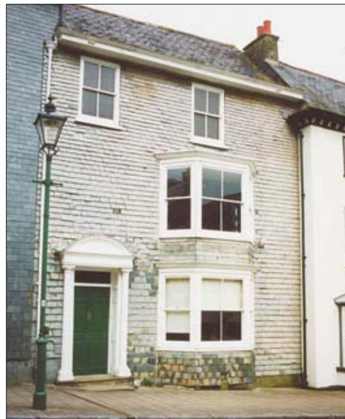
Slate hung elevations are indeed dispersed throughout the Area, but their number isn't especially great. Their prominent locations do, however, give the opposite impression. The most significant grouping, perhaps, is the row of five in Church Street, one of which – like at least two others in the Area - is preserved beneath a coating of paint. This one (above), however, is of particular note, both for the silver-grey colour of the slates and for the way they're fixed using random widths in diminishing courses (from bottom to top) – a traditional technique that's been carefully respected next door.
