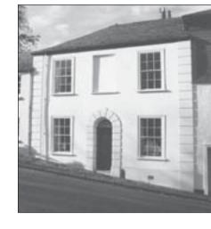
One of the more attractive of the less ornamental fronts is at 11 Cistern Street [left] which was very carefully restored in recent years when its missing rusticated quoin (at right) was reinstated. A lime-based render was used, with lime-washes over, to produce an authentic and unmistakable 'softly weathered' appearance.
