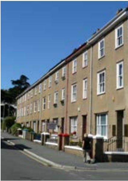
Type 2 buildings, Victoria Road
