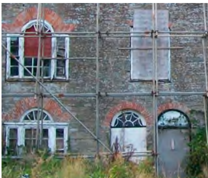
Alston Farm House, Marlborough
