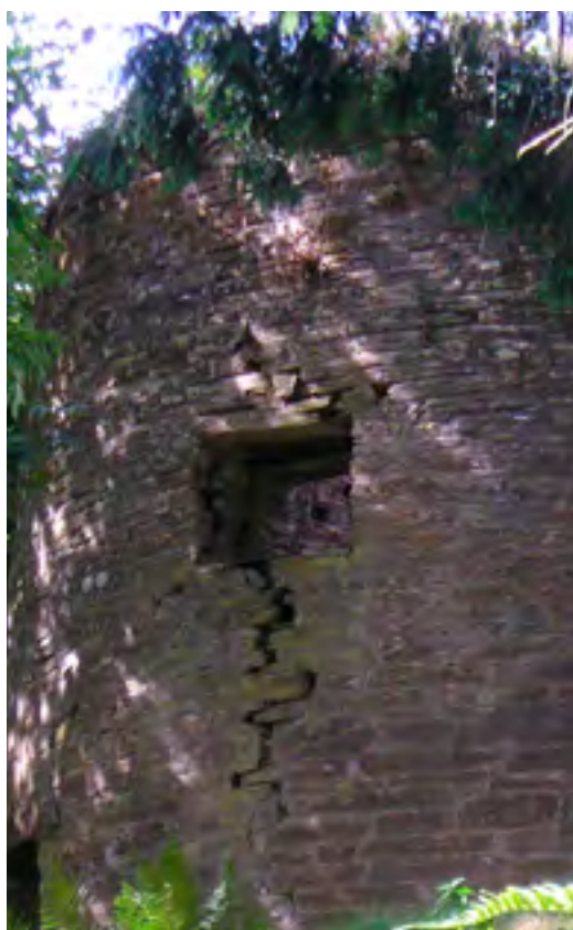
Dovecote at Bucklands-Tout-Saints Hotel
