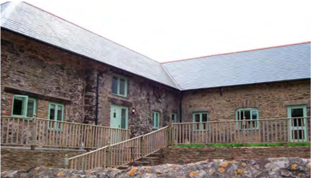
Shippen North West of Langdon Barton ( above ): Now known as White Dove Cottage, this grade II listed property was built late 18th Century early 19th Century and was originally used as an agricultural barn. The property fell into disuse mid 19th Century. A detailed scheme was agreed in the early part of 2007 to convert the shippon into a single dwelling. Works to the shippon are complete.
