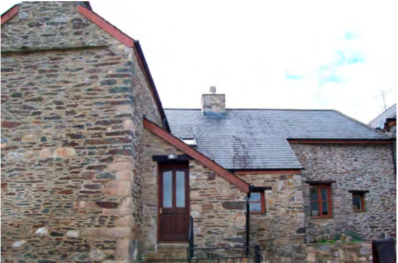
The Old Longhouse ( above ): Built in early 17th Century, this grade II listed property was originally the main farm house for the holding. A detailed scheme was agreed in 2003 to reinstate the farmhouse as a dwelling. Works to The Old Longhouse are complete.
